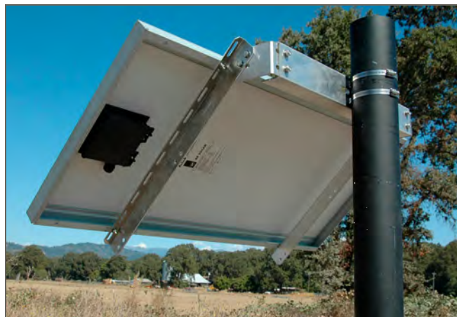
Figure 17: Solar panel mounting bracket
