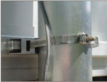
Figure 7: Sign Secured to a Pole with Banding Strap
